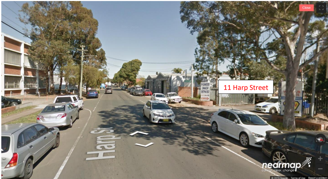
Figure 7: Existing Ausgrid Overhead Electrical Network
